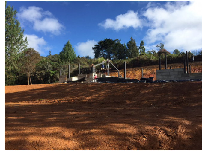
Walls at prefab house- Santa Elena
